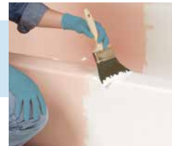
Brush: Apply in THIN, EVEN coats starting at top of surface and working down.
