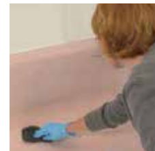
After you rinse surface with clean water and dry it with a paper towel or chamois, scour the entire surface with steel wool or sand paper.
